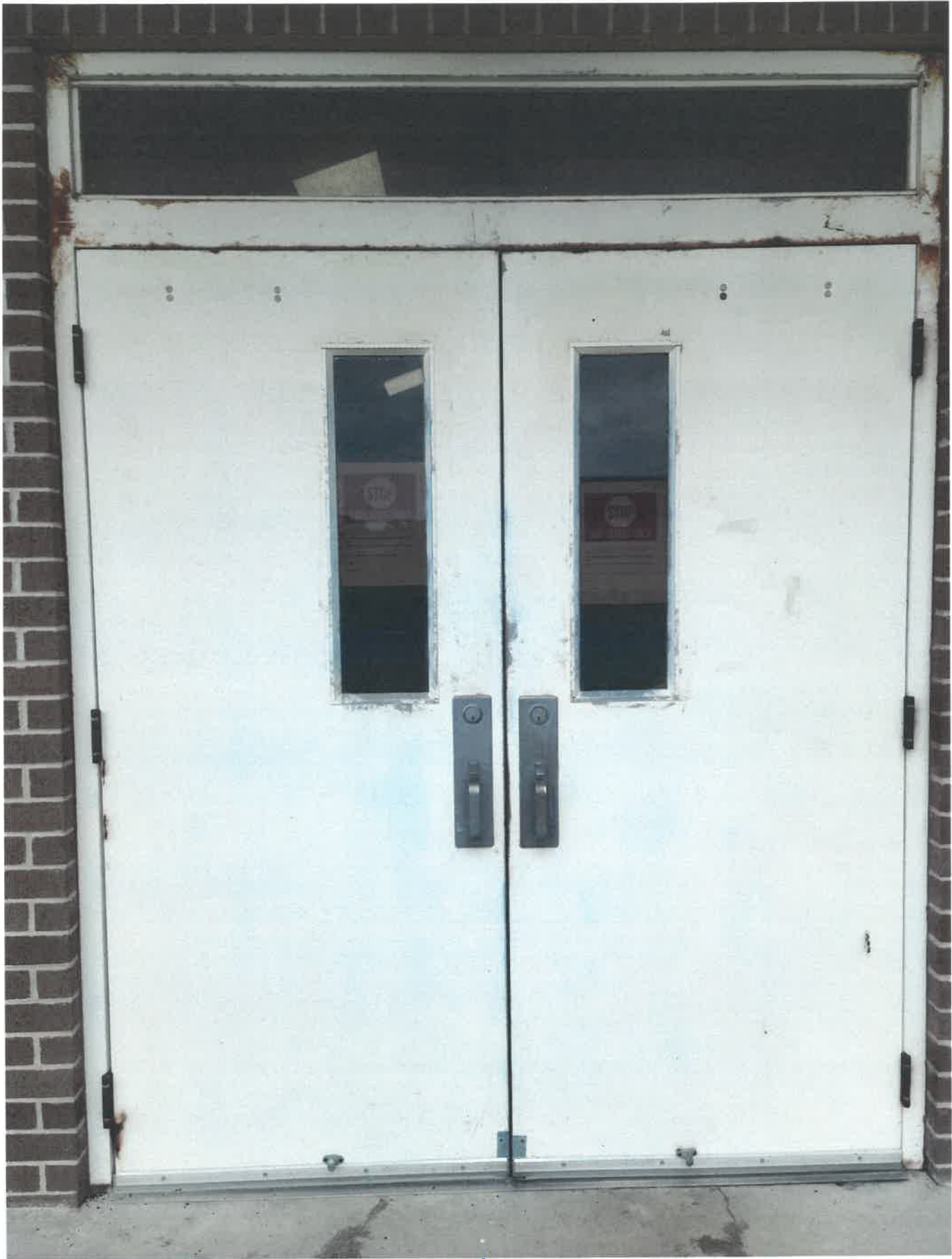
South Exterior Entrance to Dining Room
