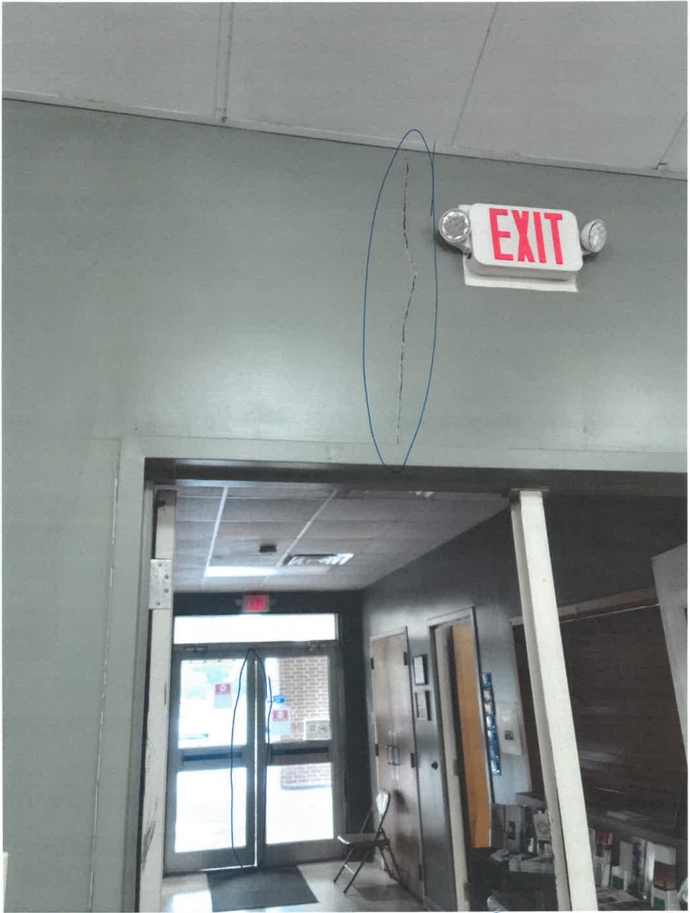
Dining Room looking to front entrance
